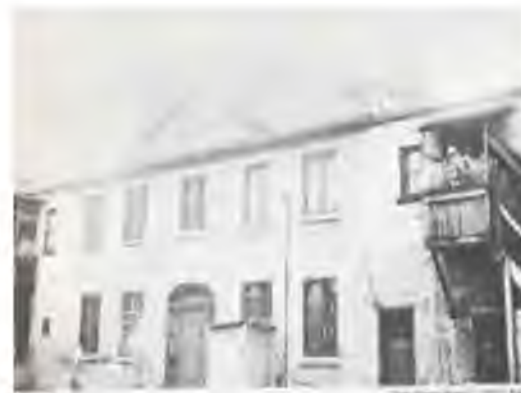
The Sparks home – built c1830
